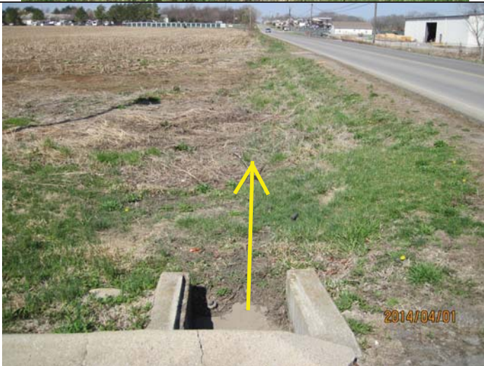
Outlet of second 18" CMP. Drainage continues West a short distance before the channel disappears in an agricultural field adjacent to Tylertown Road.
