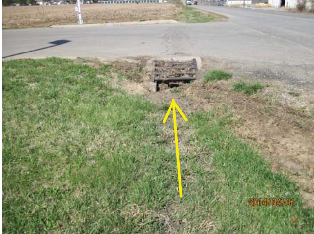
View West along Tylertown drive, at entrance to a second 18" CMP under private drive of gas station.
