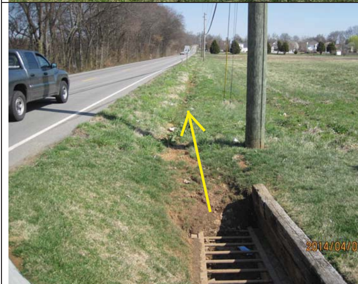
Outlet of 24" RCP under private drive. Roadside drainage continues northward along SR-48 until the channel disappears in the adjacent field.
