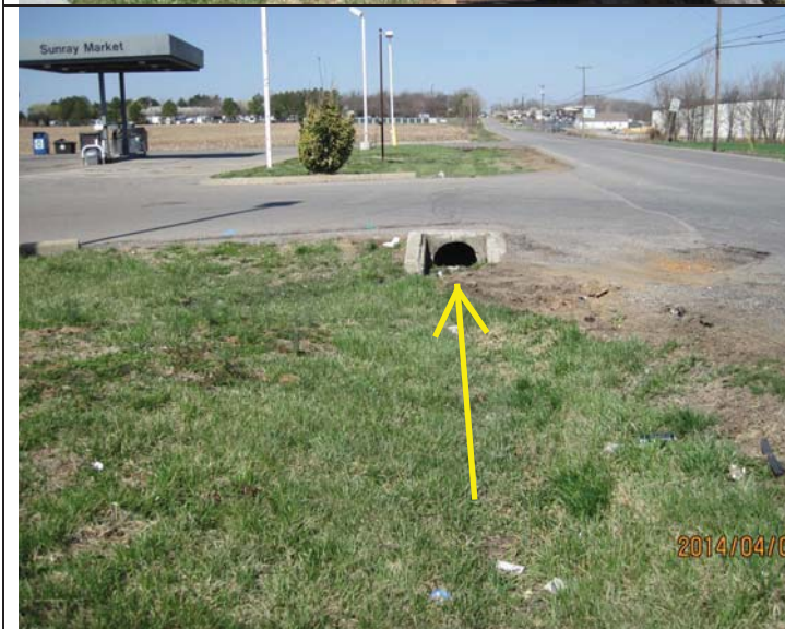
SW Corner of Project. Roadside drainage flows West along Tylertown Road and through an existing, 18" CMP under a private driveway (gas station).
