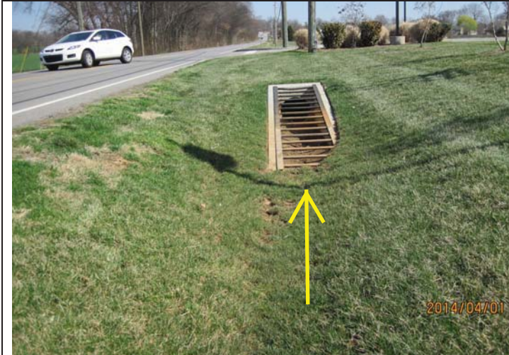
Entrance to 24" RCP under private drive. Water flows northward through this pipe and continues along SR-48.
